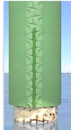
Step: 2 Insert 1 st locking key and tap it down one pitch until the key reaches the stop
